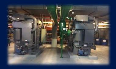
Supply, Installation and Testing & Commissioning of 4 nos. Water Cooled Centrifugal Chillers 550 TR capacity each (TOTAL 2,200 TR)
